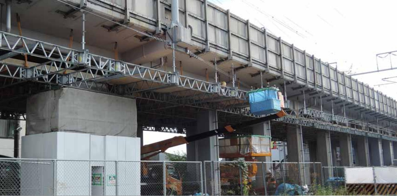
“We needed a temporary floor, which could cantilever out to safely reach well beyond the overhead structure. The QuikDeck platform is about 50-feet wide. This is key.”
