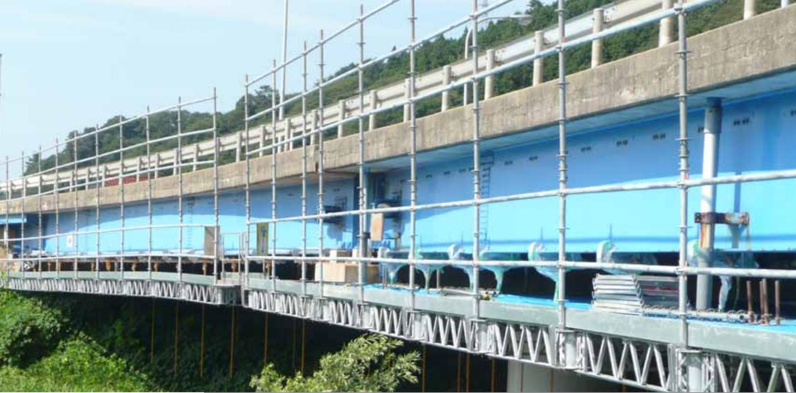
Another benefit is its fundamental strength. Depending on configuration and the spacing of suspension chains, QuikDeck can handle loads from 25 psf (pounds per square foot) to more than 75 psf.
