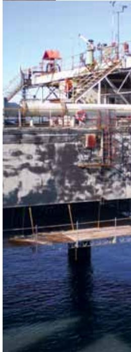
**Photos (from top to bottom):** The QuikDeck® Suspended Access System is assembled underneath the oil platform; Crews in the process of erecting QuikDeck®.
