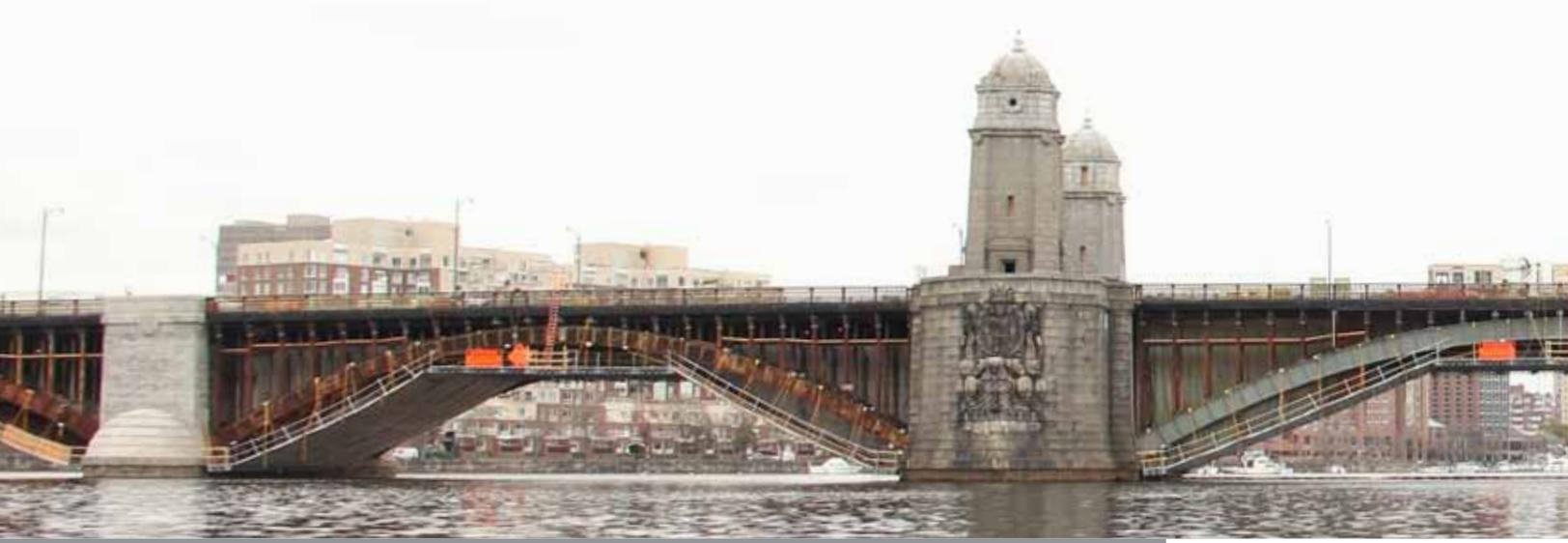
The traditional solution to bridge access involves corrugated steel decking or chain link fence supported on cables suspended from structural members. However, steel decking can become slippery when wet. It also flexes, and blasting media can be difficult to remove from the valleys. Chain link fence often induces a sense of vertigo, and the platform is not particularly stable. Neither provides a good option for material movement.
