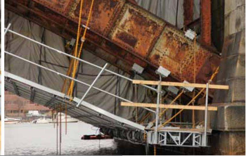
designed suspension brackets that accommodated Safway's QuikShield as well as QuikDeck. These brackets prevented the beam clamp assembly from slipping down the arch, which would have occurred with a standard clamp.
